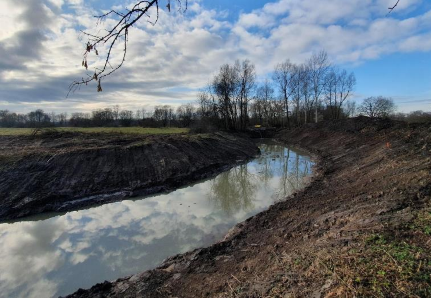
modeling of the Orlice River channel respecting the original morphology
